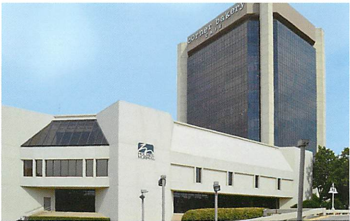
4-Level Purpose-Built Data and Technology Center
