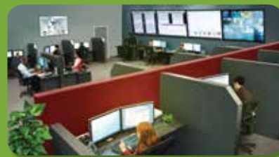
Network Operations Center (NOC)
